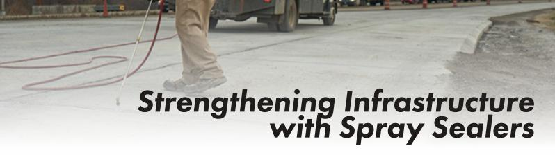
**SPRAY SEALERS CAN BE A VITAL COMPONENT** in concrete pavement preservation (CPP) due to their role in extending the lifespan and maintaining the integrity of concrete surfaces.
