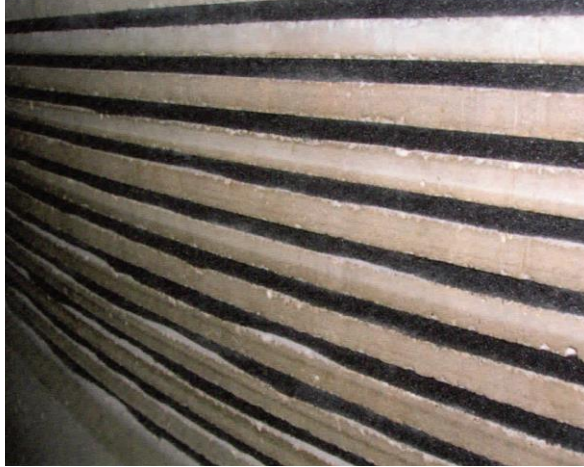
Foam Inserts Installed in Pavement
