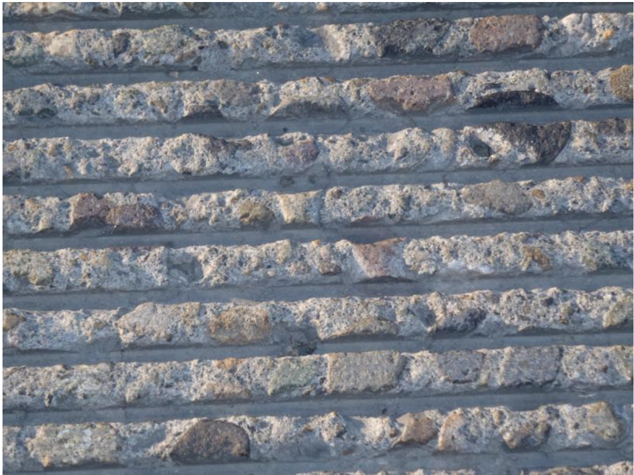
Figure 25 Apparent Attrition of NGCS Surface from Studded Tire Damage
