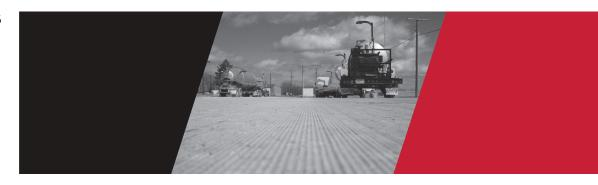
**CONVENTIONAL DIAMOND GRINDING (CDG)** is often used to create the smoothest and safest pavements available today. It is appropriate for both new construction and existing pavement and can be performed at any time during a pavement's life.
