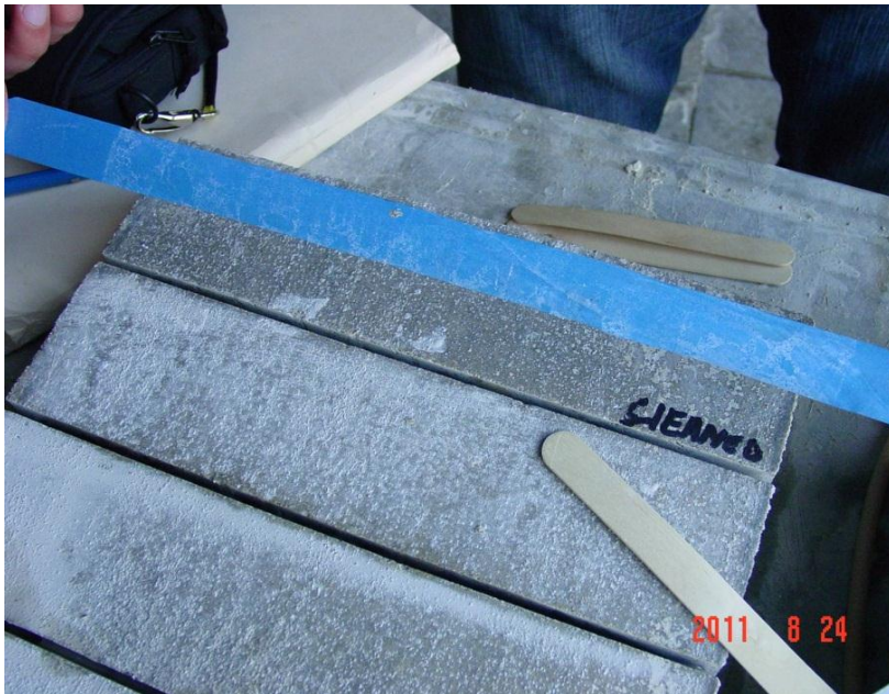
Figure 14. Blue painters tape test result on cleaned joint.
