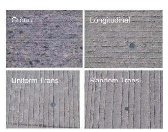
Fig. 1: Primary types of concrete surface texturing – vehicle travel from left to right.
