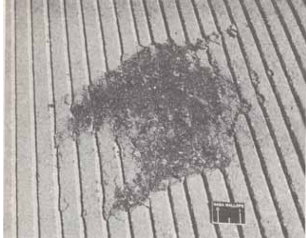
Figure 5 Damaged grooves by Convair 990 during 180 ° turns at Wallops Facility (3)
