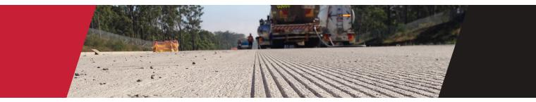
NASA did extensive research in the 1960s and 70s on aircraft hydroplaning and concluded that transverse grooving was superior to longitudinal grooving on runways for water removal and hence hydroplaning prevention. Simply put, the transverse direction has a shorter path for the water to travel to get out from beneath the tire contact patch. Full scale testing with actual aircraft was conducted in that effort.
