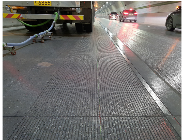
NGCS being installed in Korea's long tunnels, courtesy Hexacon
