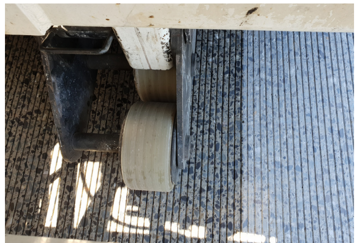
NGCS being installed in New South Wales
