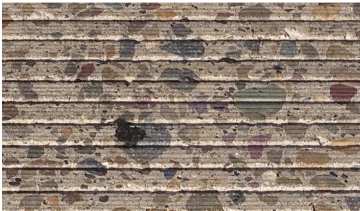
NGCS installed on I 5 in San Diego, California
