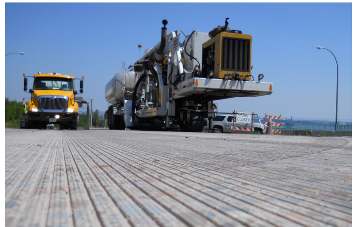
NGCS pavement installed in Duluth, Minnesota
