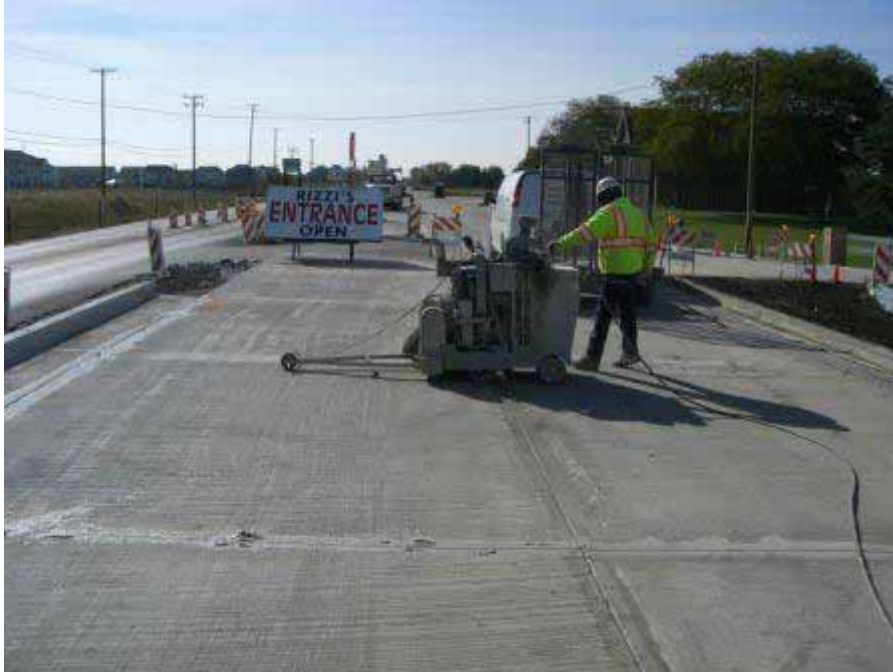
Initial Saw Cut
