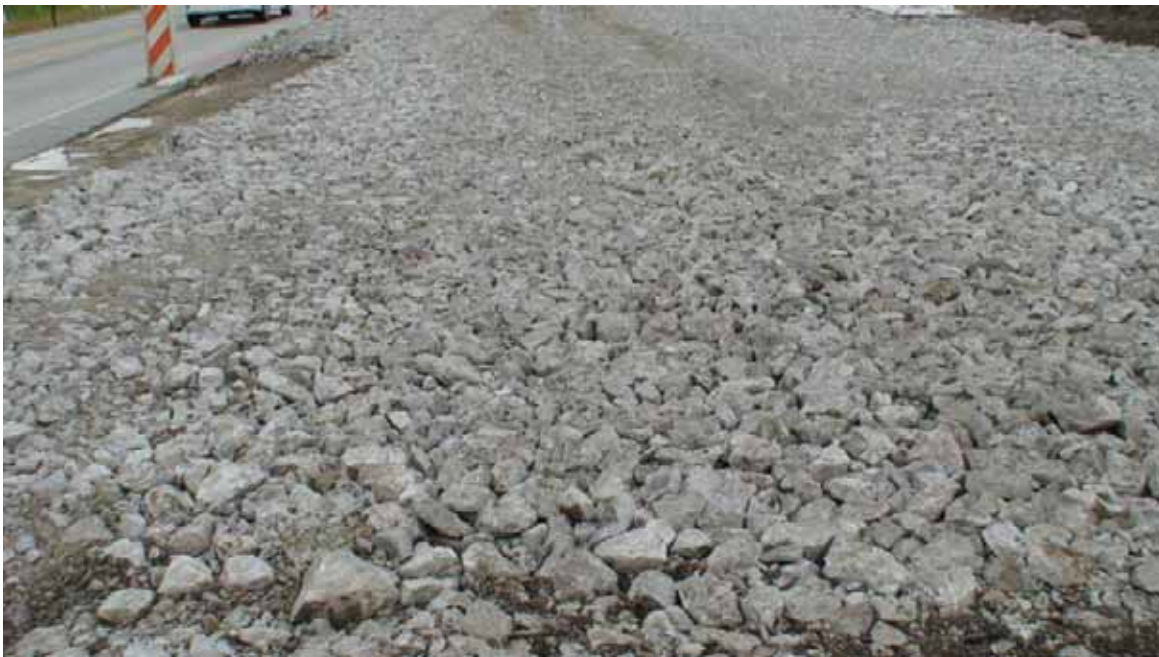
Figure 3 Six Inch Top Size Crushed Concrete Base
