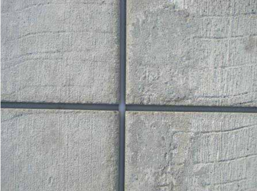
Backer Rod Installed in Mainline
