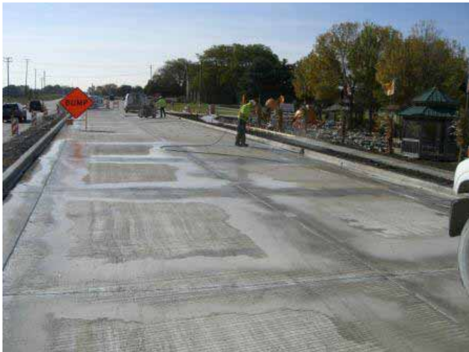
Widening Cut and Power Washing
