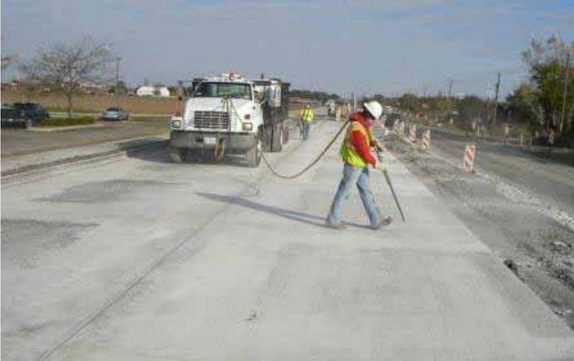
Blowing Out Debris In Advance of Sealant Installation
