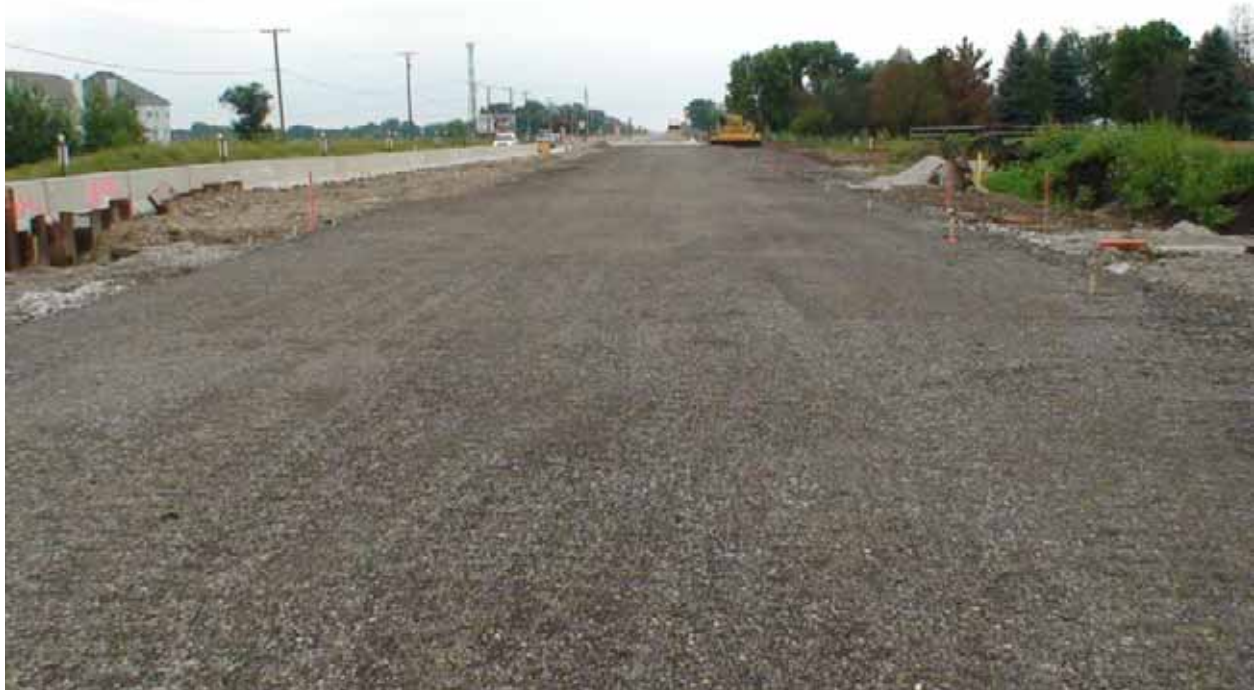
Figure 4 Three Inch Thick AC Millings Plating Crushed Concrete
