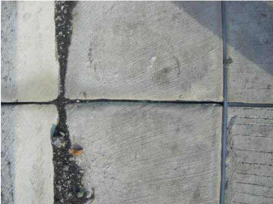
Backer Rod Installed in Curb Joint
