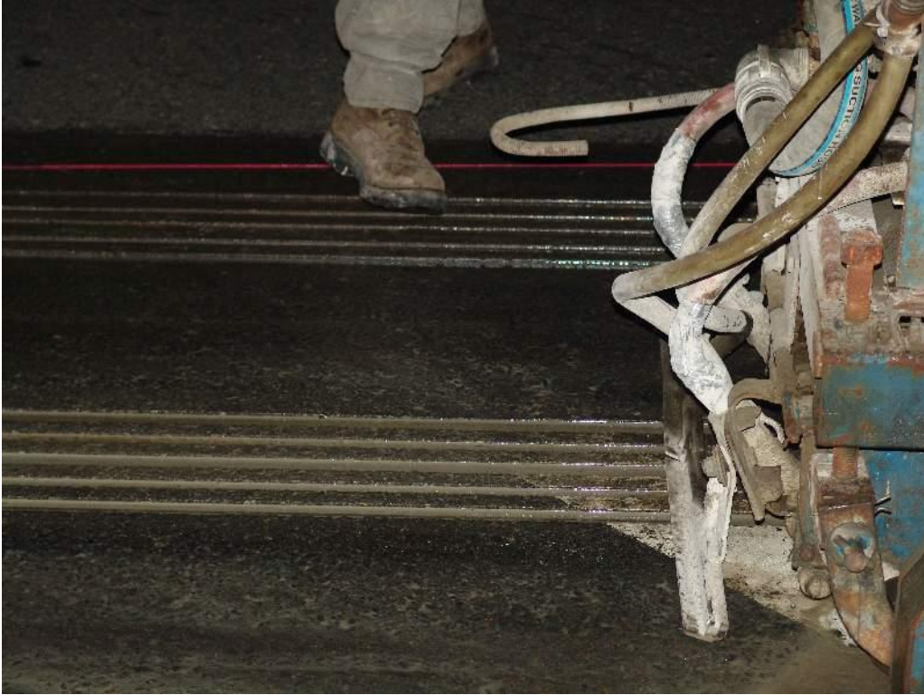
Figure 5 – Groove Cutting Equipment and Process
