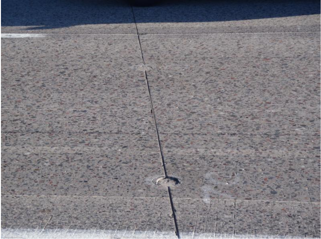
Figure 4-7 6" Core Hole Depression
