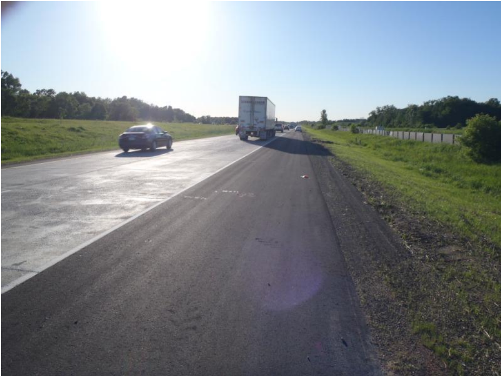
Figure 1-2 Overview of Exposed Aggregate Test Section
