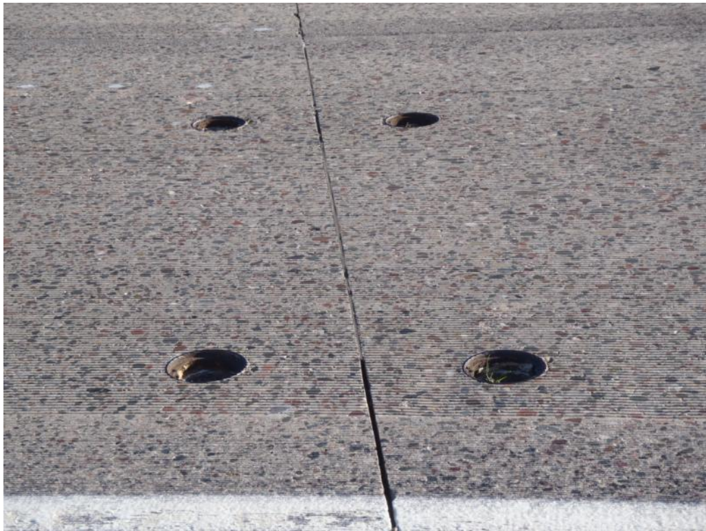
Figure 4-4 Hand Holes in Pavement
