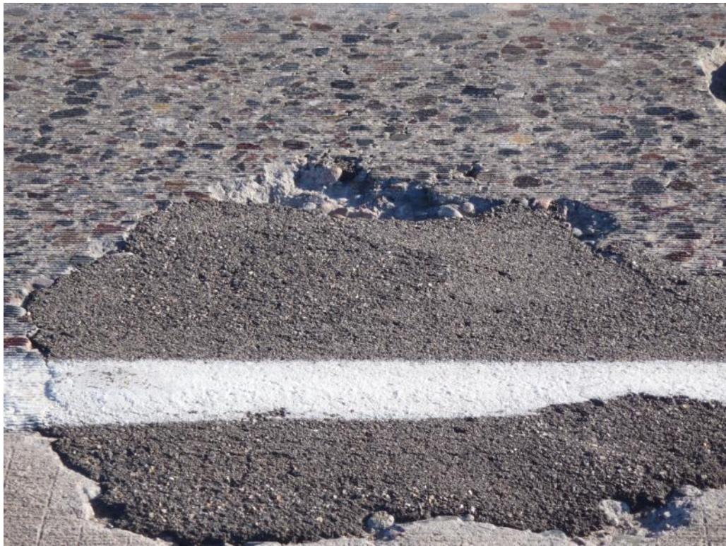
Figure 3-6 Pot Hole Repair at Edge of Pavement
