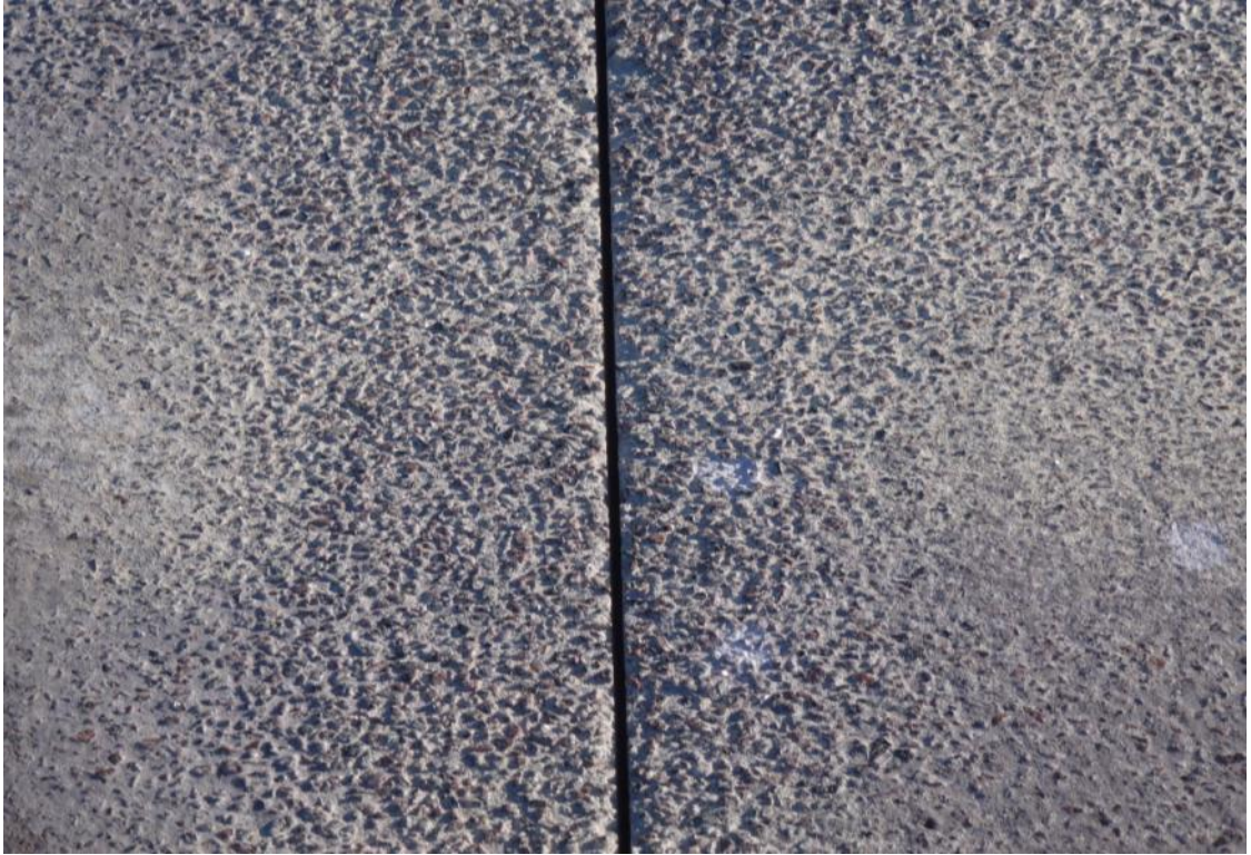
Figure 1-3 Close up of Exposed Aggregate Texture and Transverse Joint
