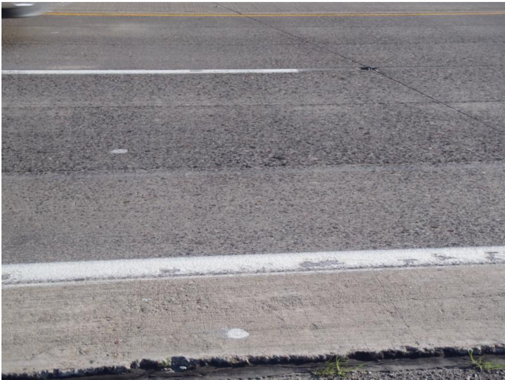
Figure 3-4 Texture in Outside Pass Appears Different
