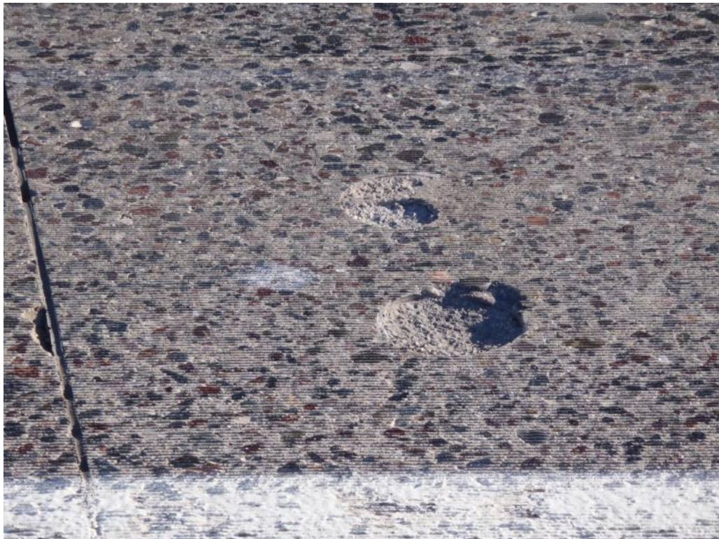
Figure 3-2 6" Core Hole Repairs
