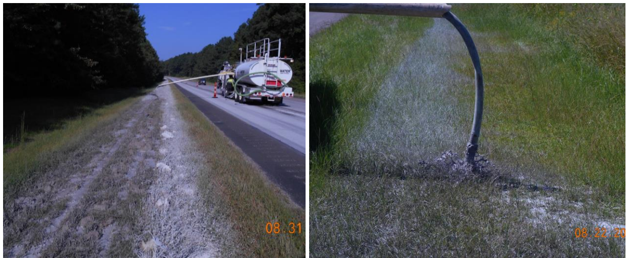
Figure 5. DGS on furrowed shoulder (left) and DGS discharge from grinding machine (right).
