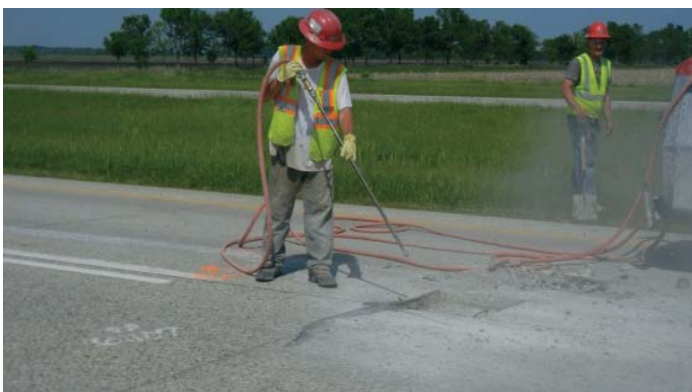
Figure 33. Air blasting to remove loose debris
