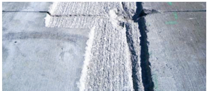
Figure 19. Type 2A joint milling
