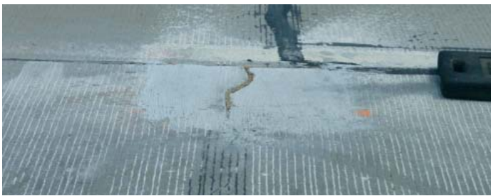
Figure 49. Completed Type 1 crack repair
