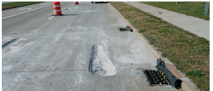
Figure 18. Type 1 spot milling
