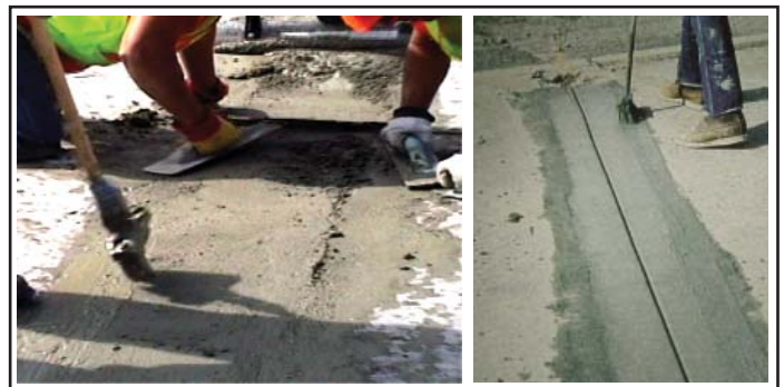
Figure 48. Placement of grout at edge of partial-depth repair
