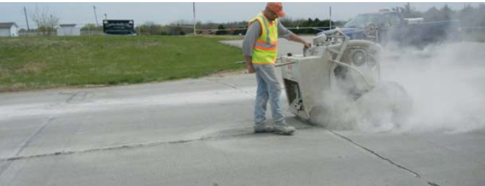
Figure 47. Sawing following tooling the joint
