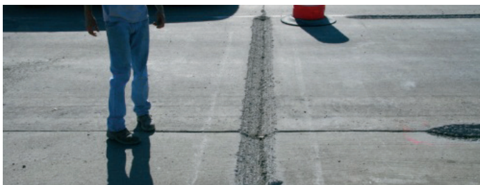
Figure 21. V-head milling (Types 1 and 2)
