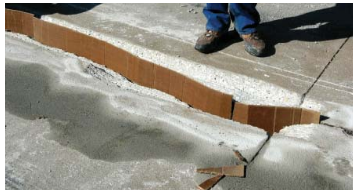
Figure 37. View of cardboard cut to fit irregular random crack
