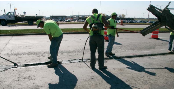
Figure 42. Consolidation of repair material for Type 2A joint repair
