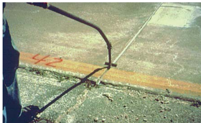
Figure 56. Joint sealing
