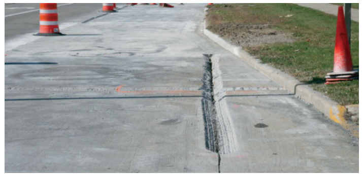
Figure 16. Milling along the joint or crack
