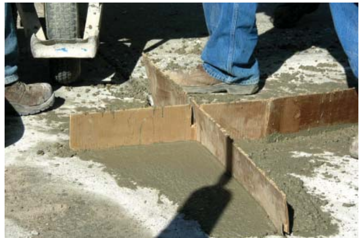
Figure 45. Concrete placement for Type 1 repair using waxed cardboard
