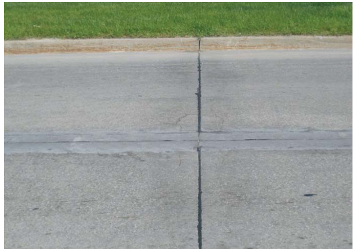
Figure 68. D crack repair
