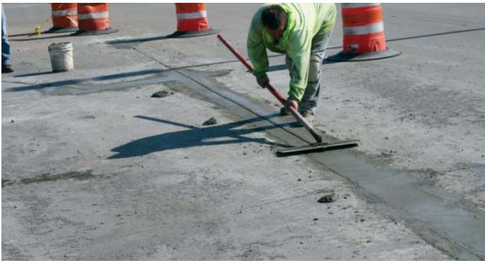
Figure 46. Tooling the joint
