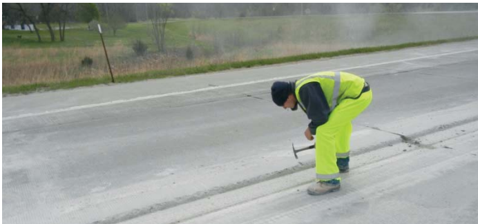
Figure 31. Sounding with hammer
