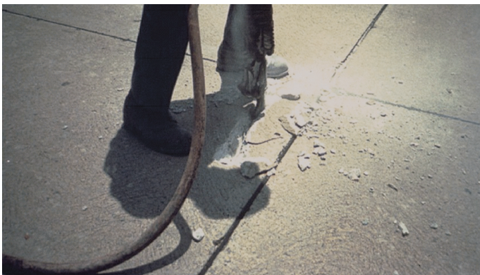
Figure 28. Type 3 repair – Removal with small jackhammer
