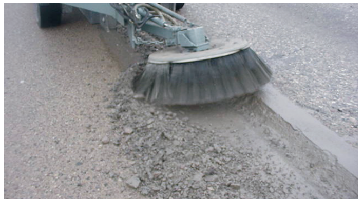
Figure 30. Sweeping loose material
