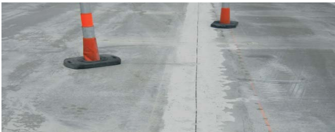
Figure 50. Completed Type 2A joint repair
