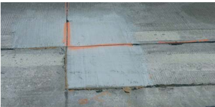
Figure 52. Completed Type 3 repair
