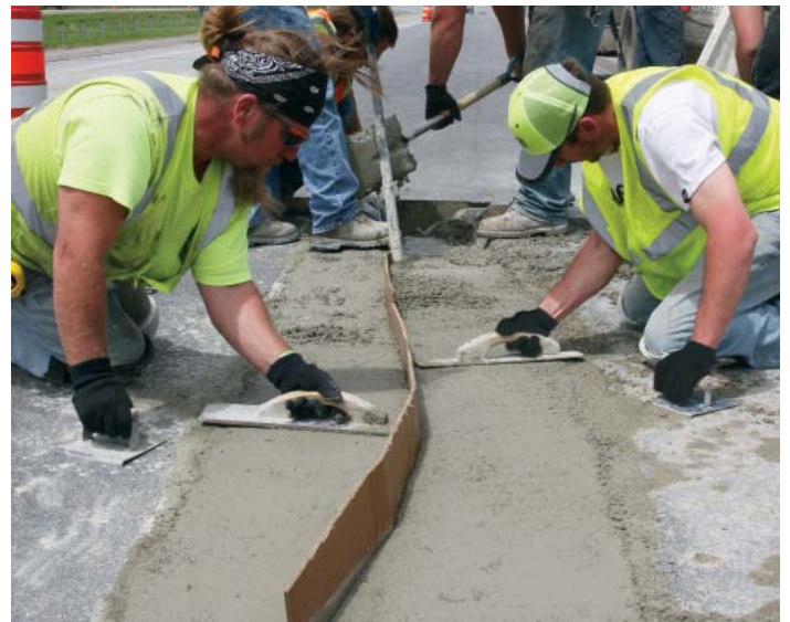
Figure 44. Troweling toward the edge of the repair
