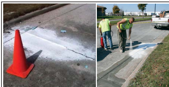
Figure 53. Curing of repair material
