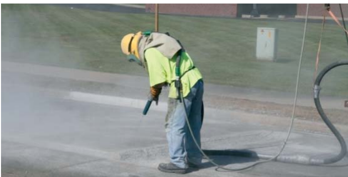
Figure 32. Sandblasting to remove loose debris
