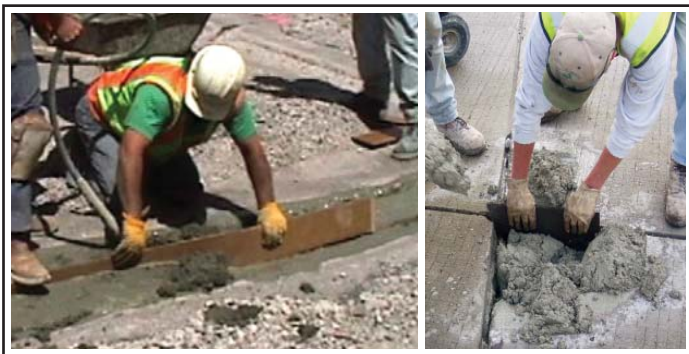
Figure 43. Concrete placement while holding waxed cardboard
