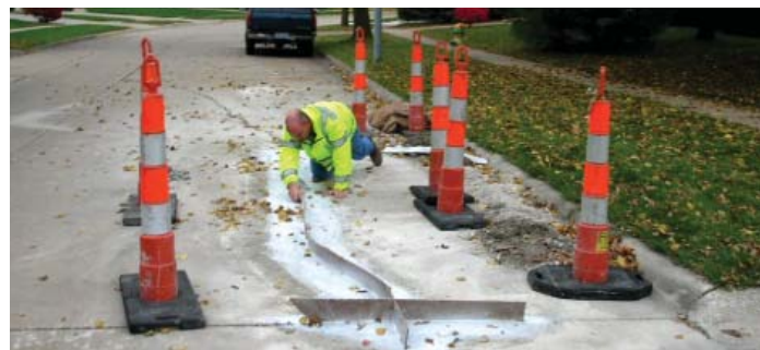
Figure 54. Cutting excess compression relief board of Type 2B crack repair
