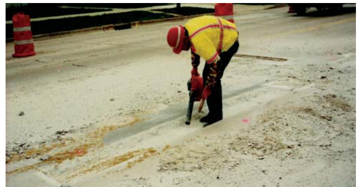
Figure 34. Using a leaf blower for final removal of any contaminants
