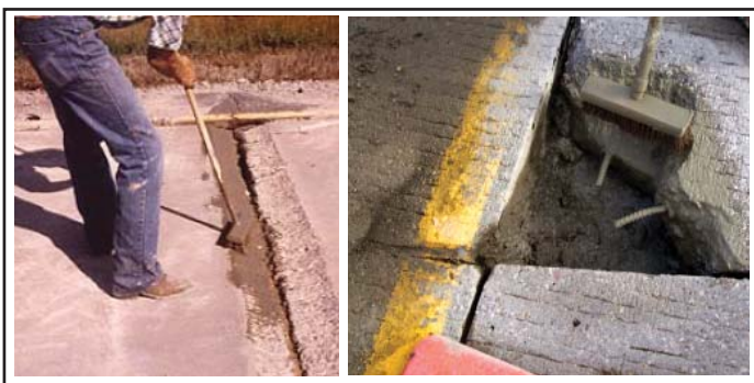
Figure 39. Placement of cement grout as bonding agent
