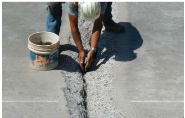
Figure 59. Proper use of sand to prevent lockup of joint
