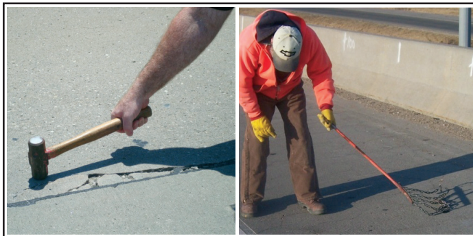
Figure 13. Sounding deteriorated concrete using a hammer (left) and steel chain (right)
