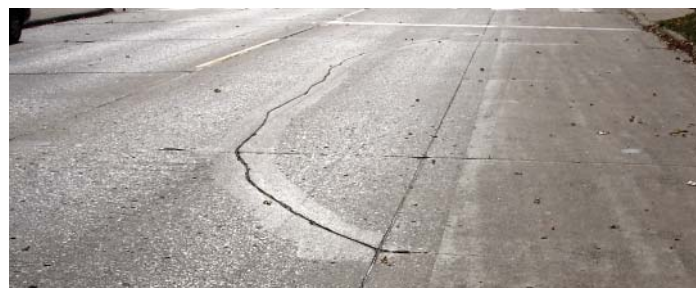
Figure 55. Diamond grinding of partial-depth patch
