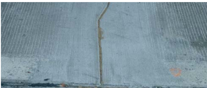
Figure 51. Completed Type 2B crack repair
