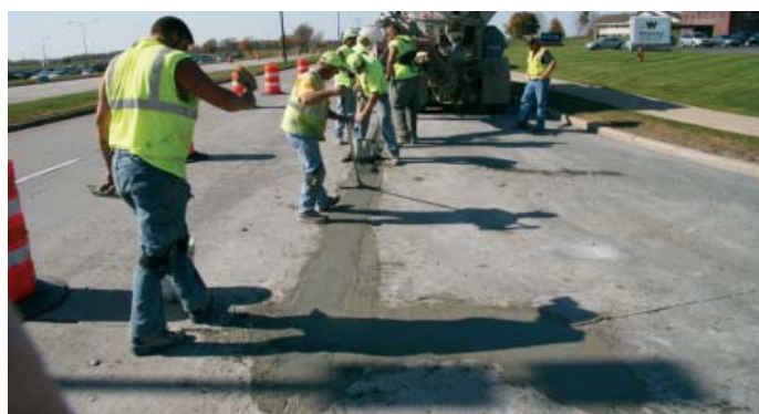
Figure 41. Placement of repair material
