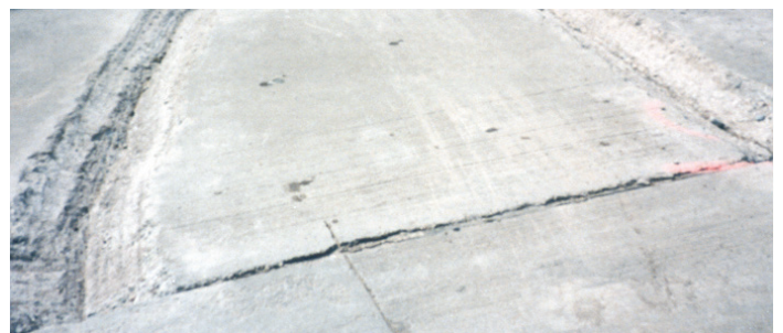
Figure 20. Type 2B crack milling
