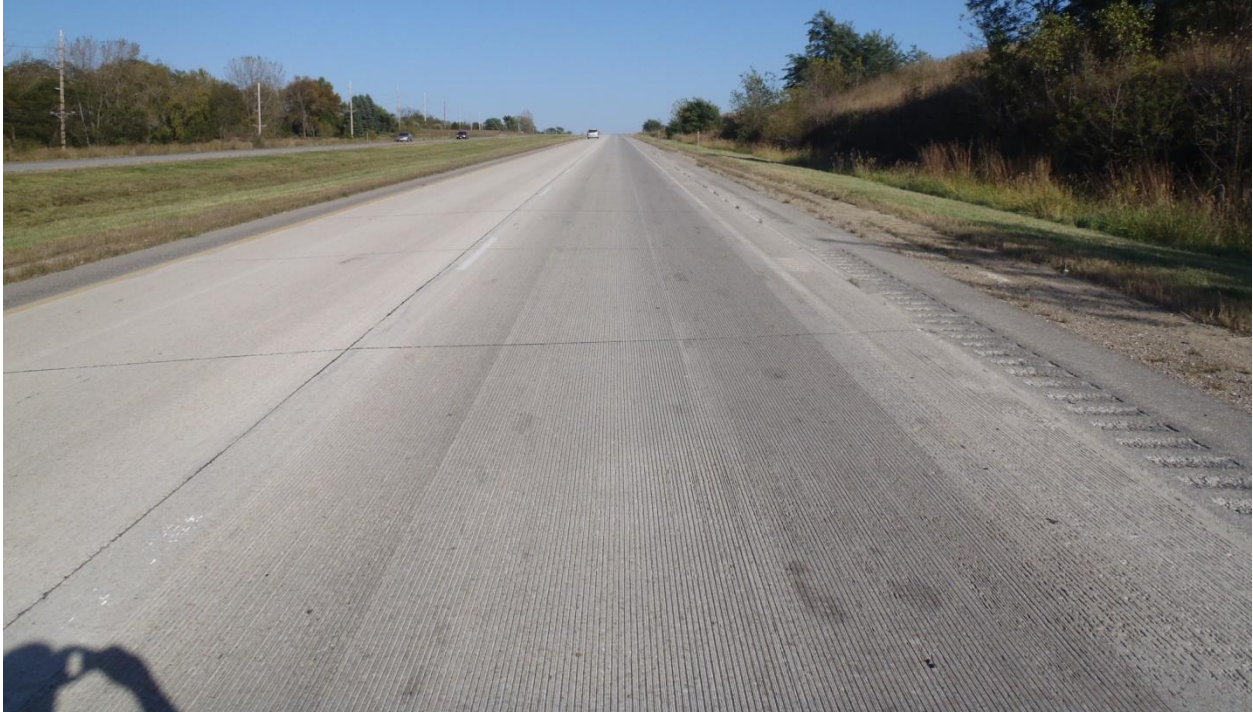
Figure 2-1 Overview of Test Section 2 for CDG with \frac{3}{4} " Groove Spacing
