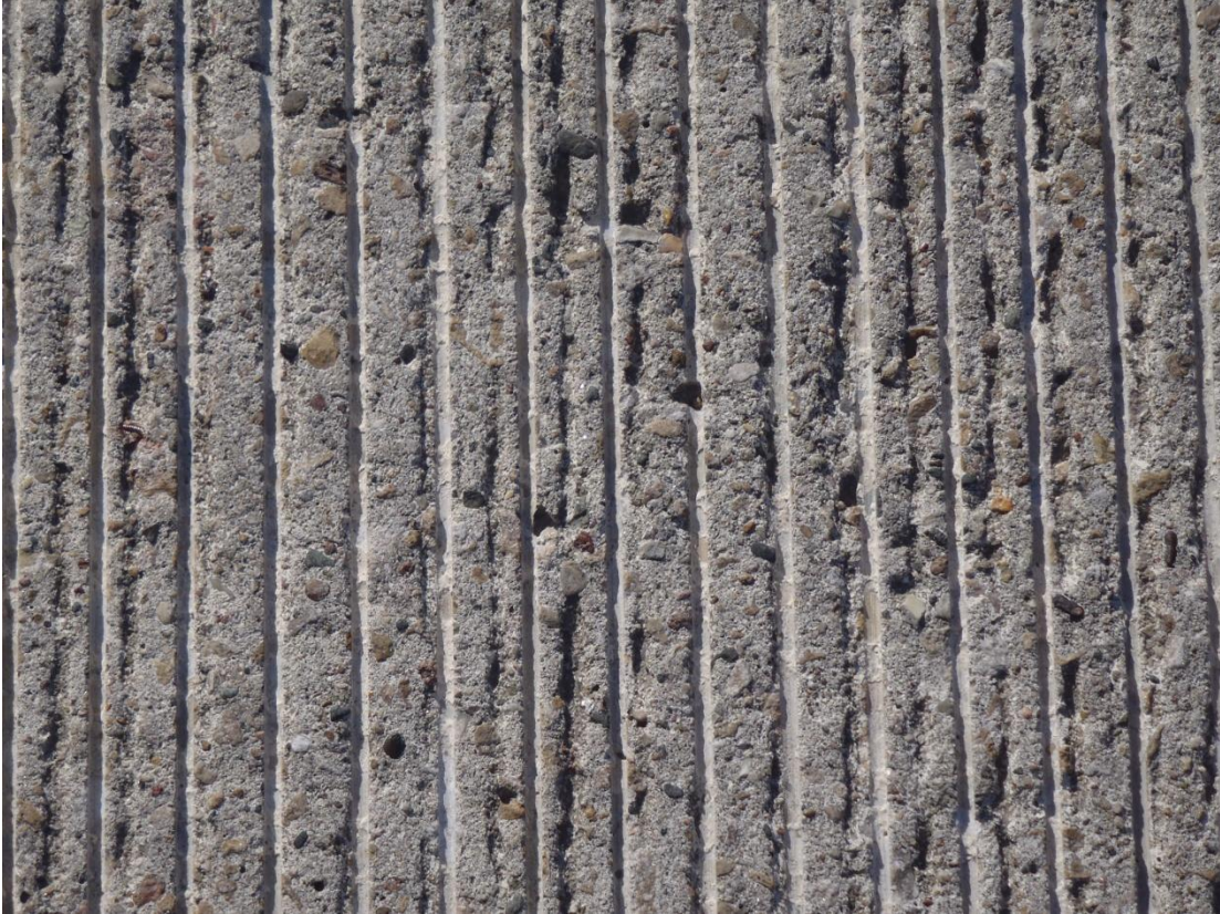
Figure 4-3 View of Aggregate Size Evident in Original Pavement
