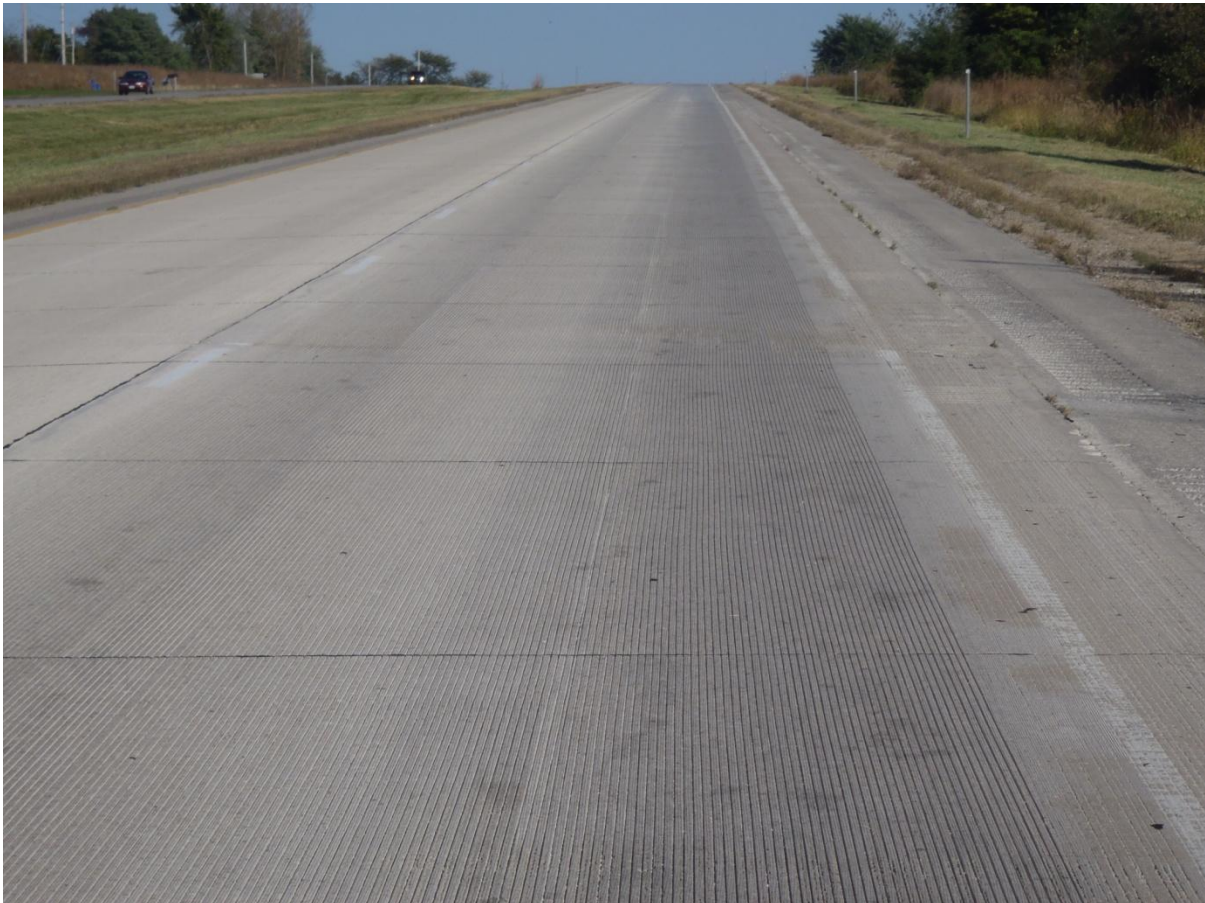
Figure 2-2 Overview of CDG with \frac{3}{4} " Grooving on Section 2
