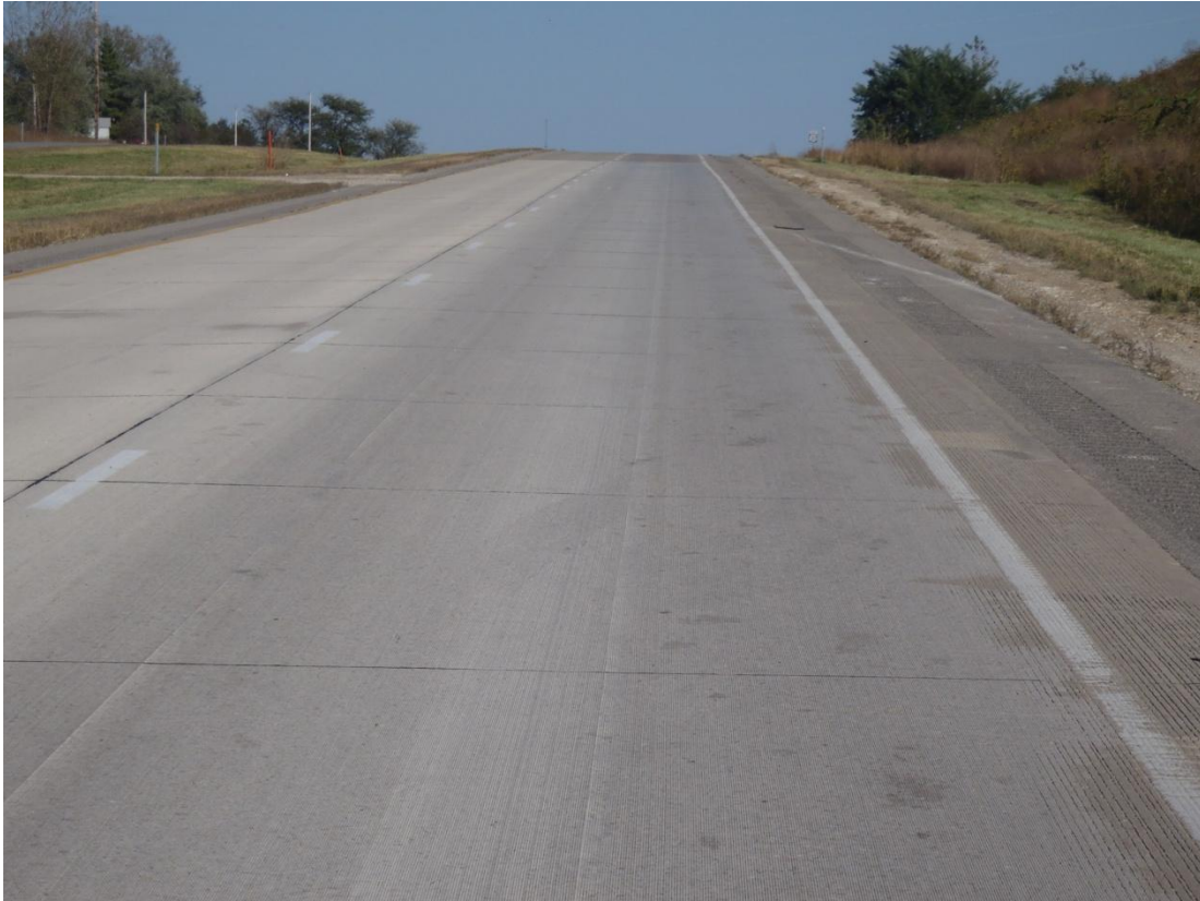
Figure 3-1 Overview Photo of CDG Test Section 3
