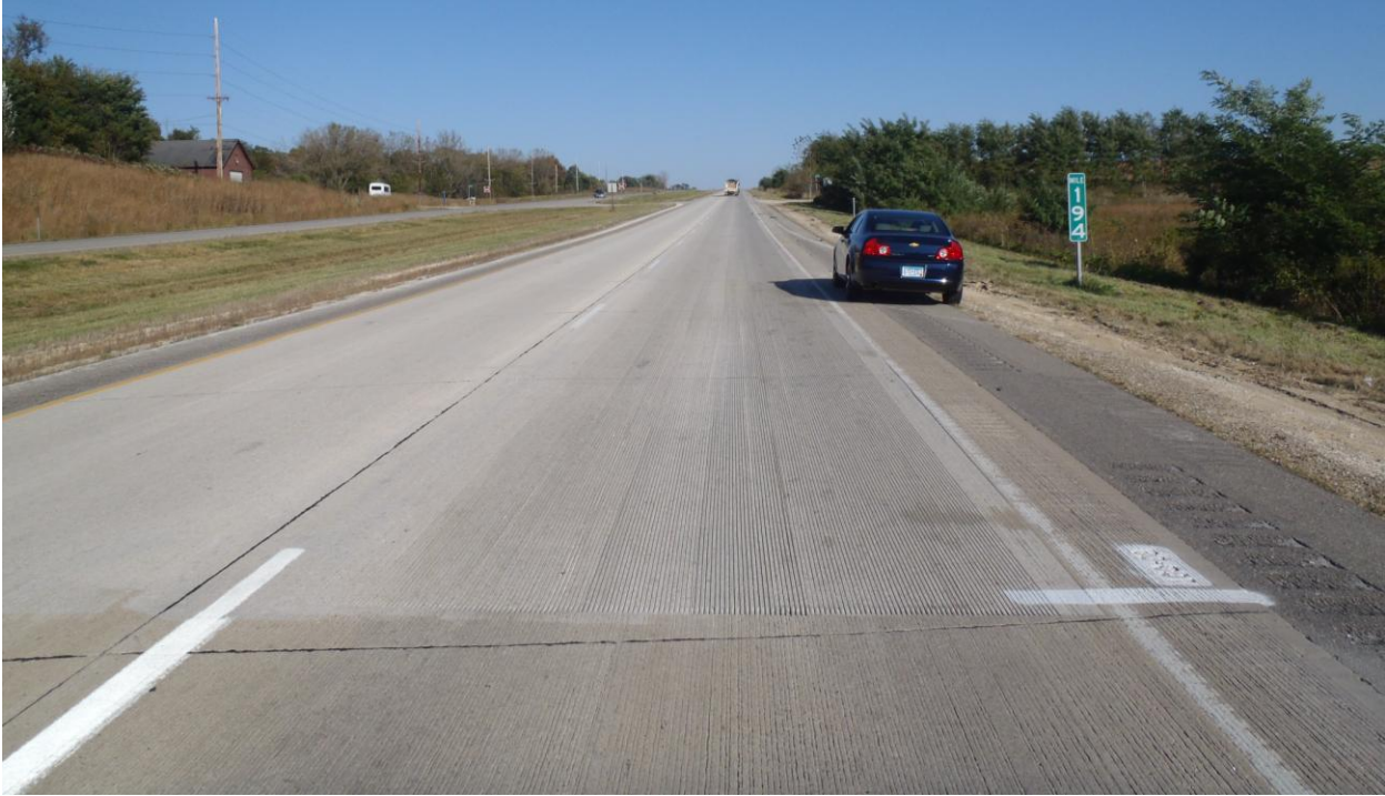
Figure 1-1 Overview Photo of Flush Ground and Grooved Test Section 1
