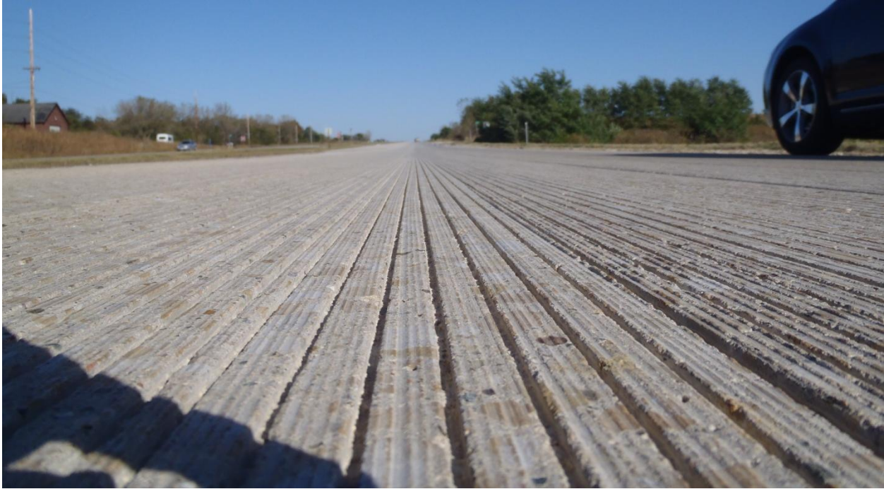
Figure 1-5 Ground Level View of Flush Ground and Grooved Texture on Section 1
