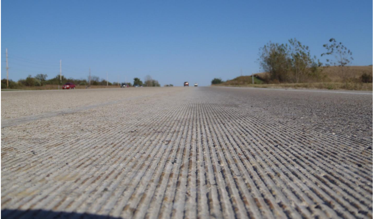
Figure 3-3 Ground Level View of CDG Texture in Section 3
