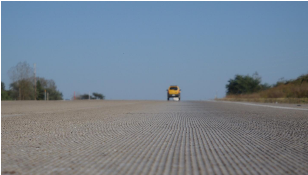
Figure 3-2 Ground Level View of CDG Texture in Section 3
