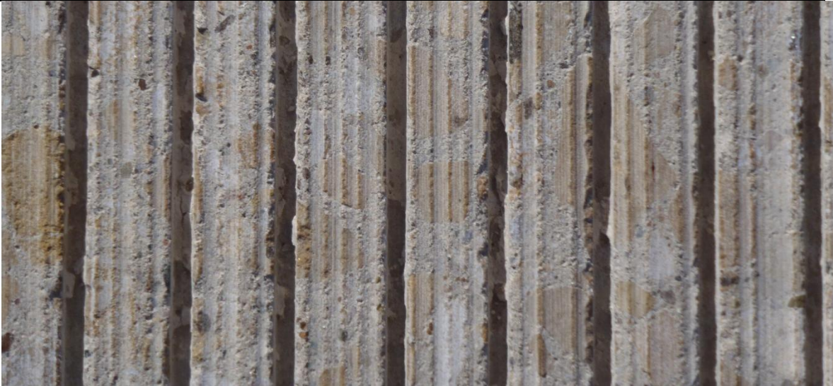
Test Section 1 Flush Grind and Groove
