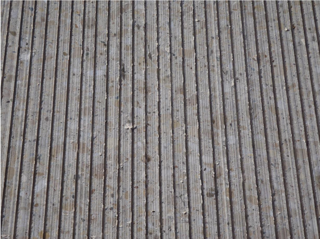
Figure 1-4 Close Up of Flush Ground and Grooved Texture on Section 1
