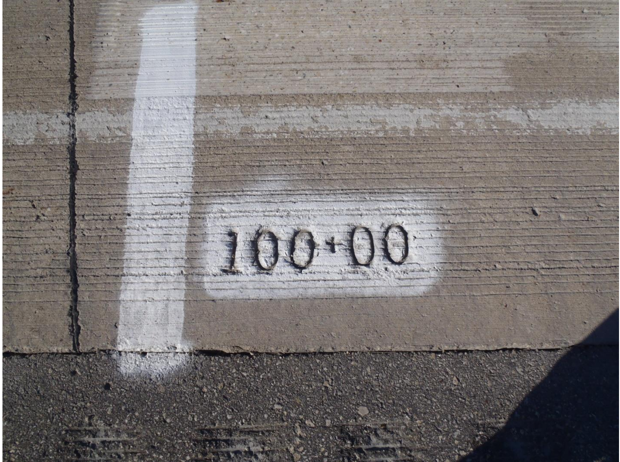
Figure 1-7 Stationing 100 Indicating Beginning of Flush Ground and Grooved Section 1
