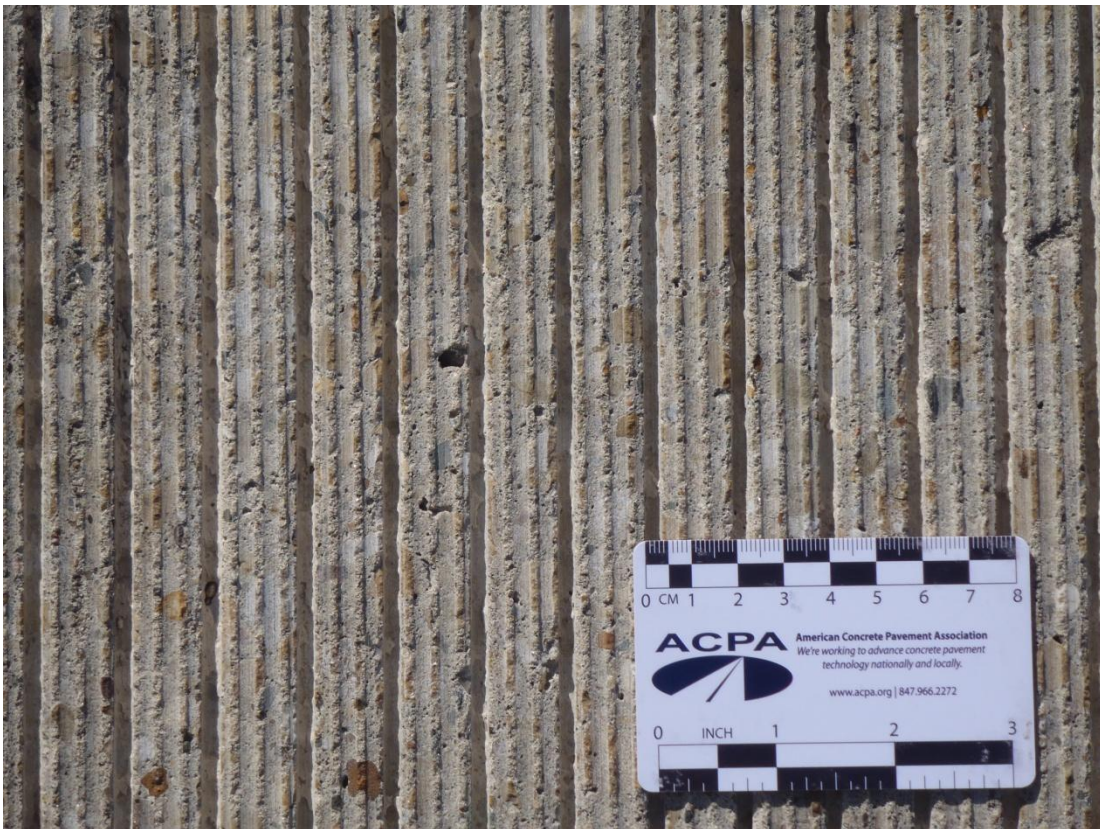
Figure 2-4 Close Up of CDG Texture with \frac{3}{4} " Groove Spacing on Section 2
