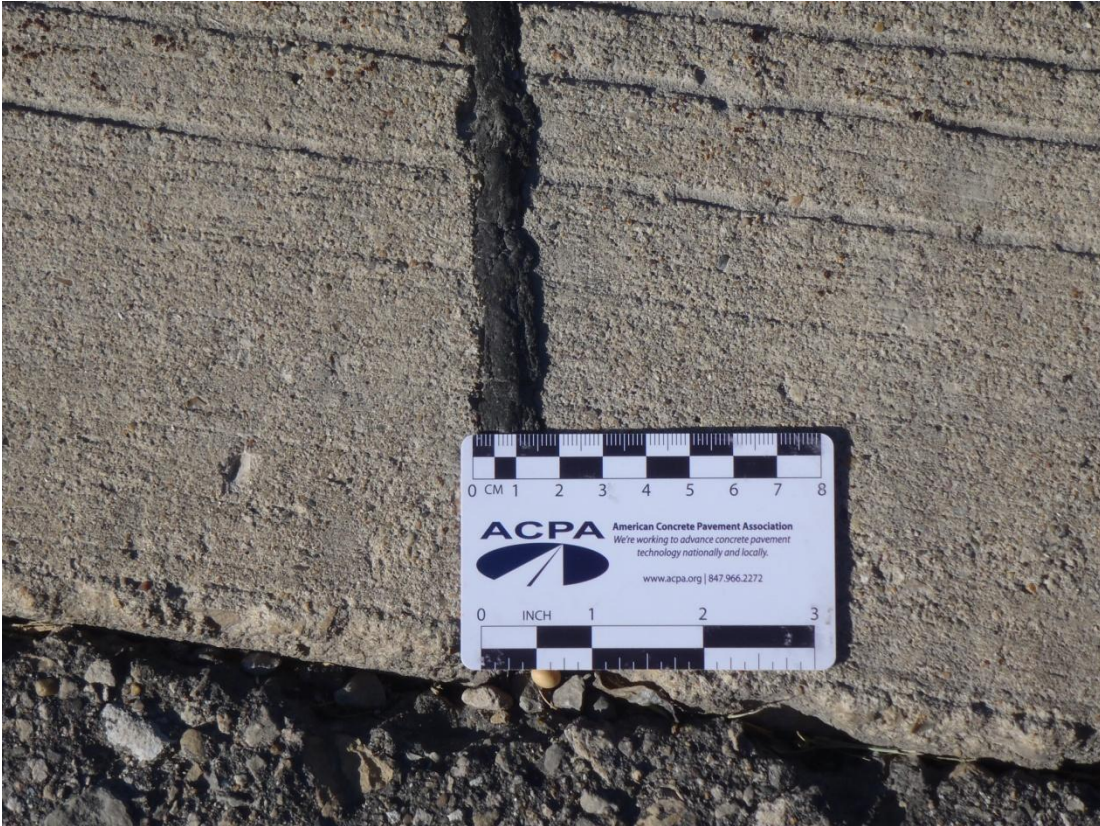
Figure 4-1 Photo of Transverse Joint Sealant on Existing US 30 EB Pavement
