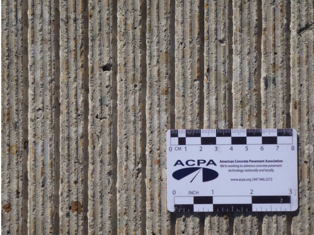
Figure 2-3 Close Up of CDG Texture with \frac{3}{4} Groove Spacing on Section 2
