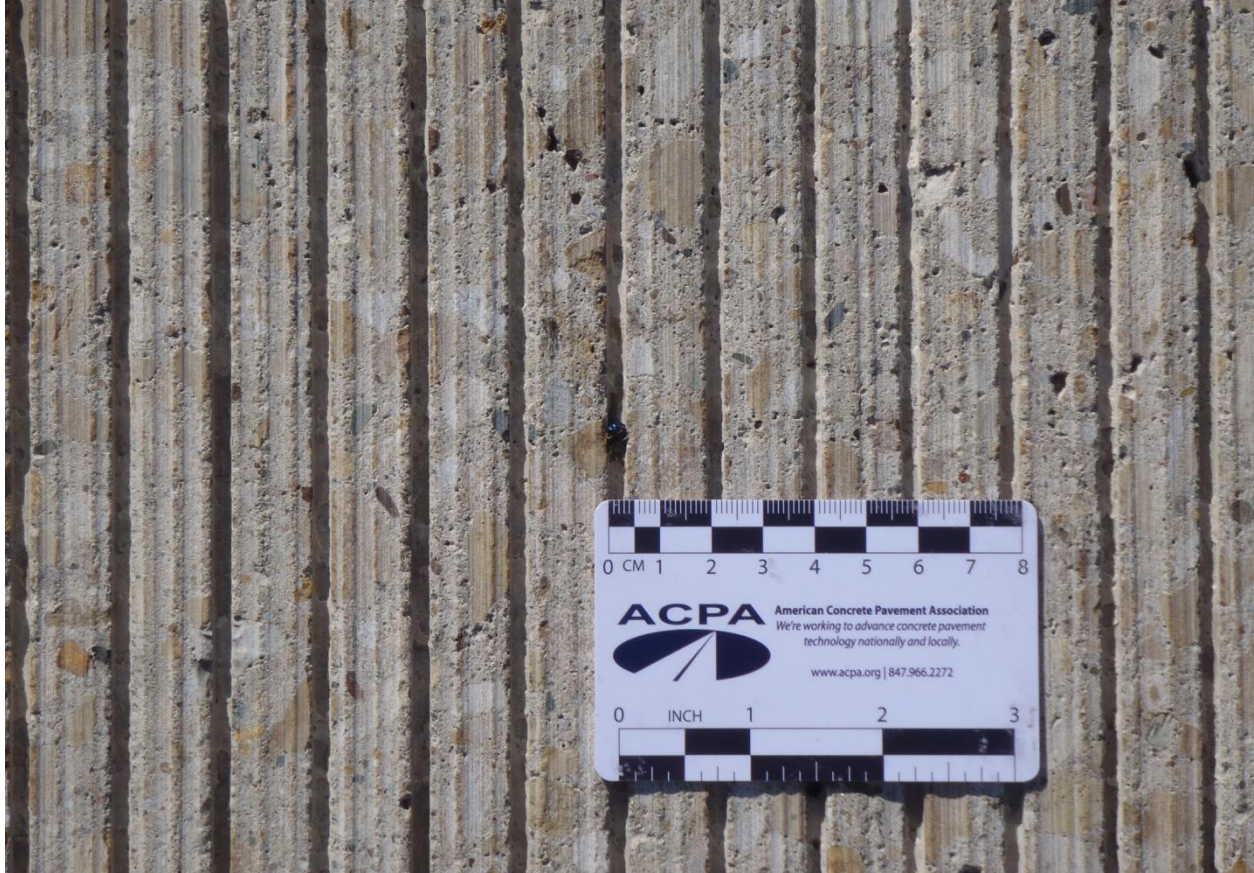
Figure 1-2 Close Up of Flush Ground and Grooved Texture in Test Section 1
