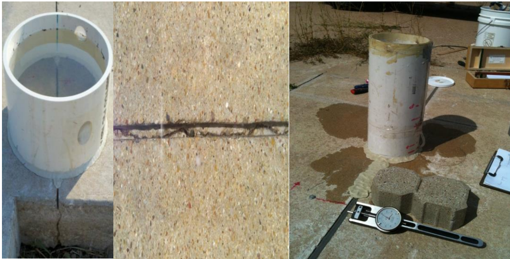
Figure 7 Flow Test on Existing Joint.
