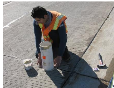
Figure 22 SR 59 Infiltration Testing (2013).
