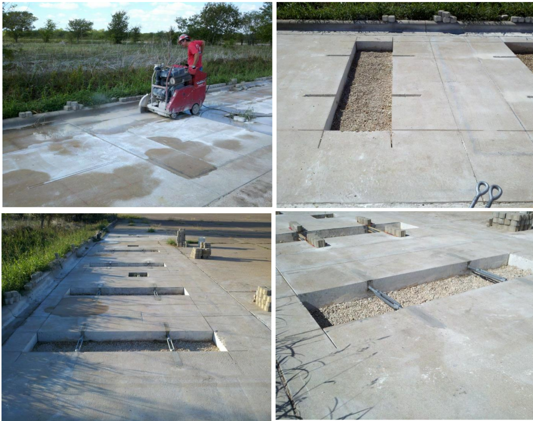
Figure 11 Installation of Movable Joint System.
