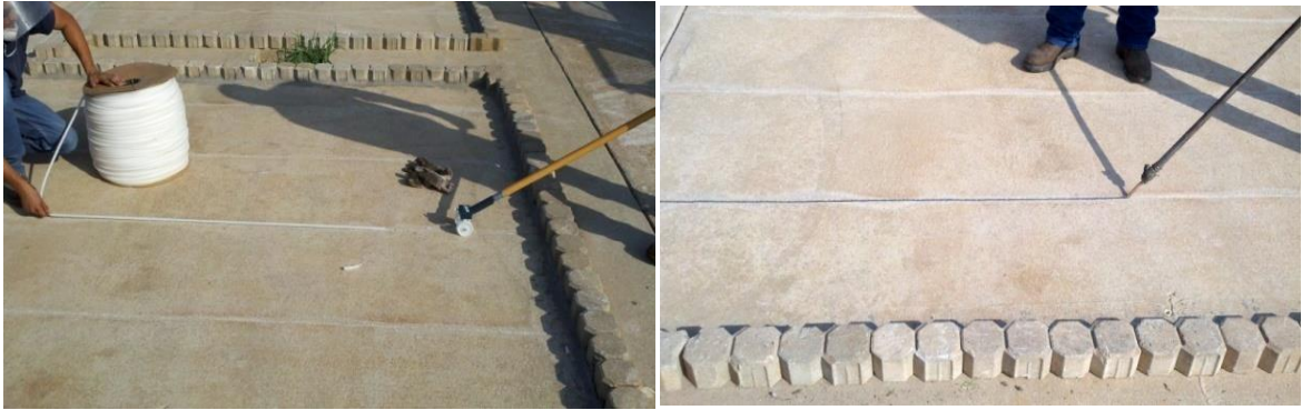
c) Backer Rod Placing
